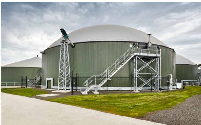
Yarra Valley Water's waste-to-energy facility converts biosolids to biogas. Image supplied by Yarra Valley Water.
