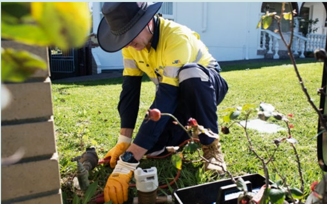
WA Water Corporation's smart meters make billing more efficient, provide information about water use and help the utility detect leaks. Image supplied by WA Water Corporation.
