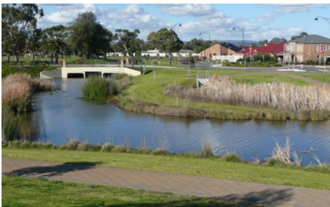
The City of Salisbury manages more than 50 constructed wetlands and treats approximately 8 gigalitres of stormwater each year. Photo of Springbank Waters, Burton, City of Salisbury. Image supplied by City of Salisbury.
