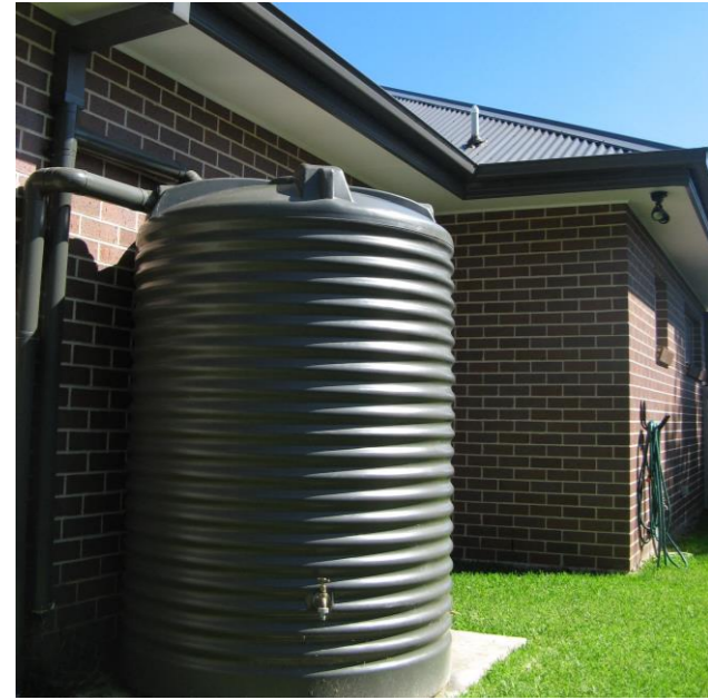
Rainwater Tanks in Perth
