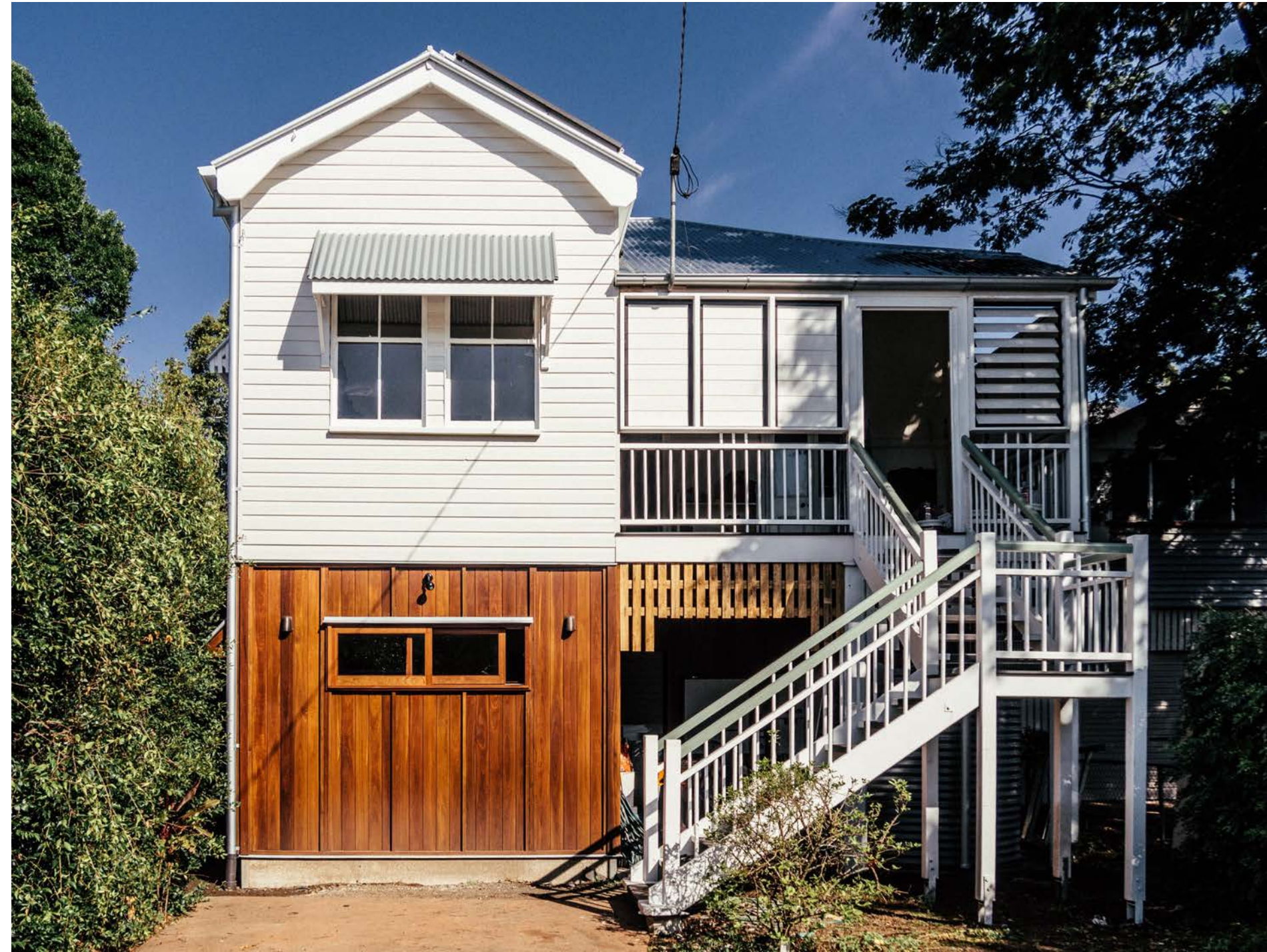
Chelmer Flood House
