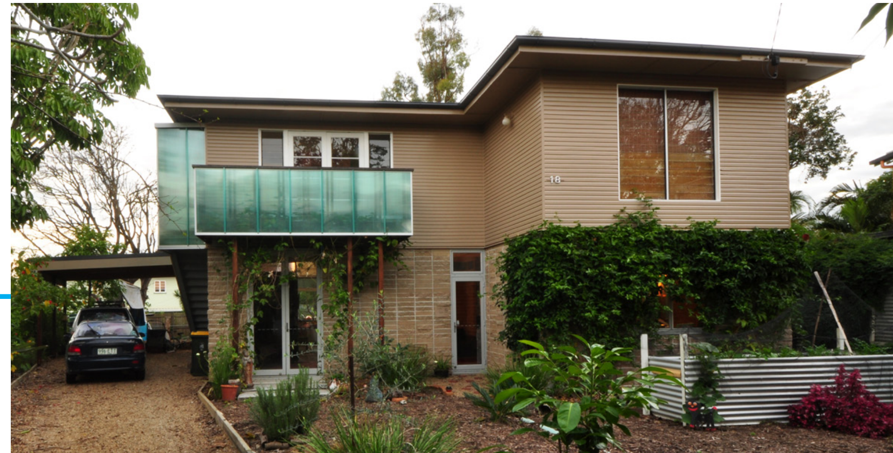
RENOVATED HOUSE JDA ©2011
