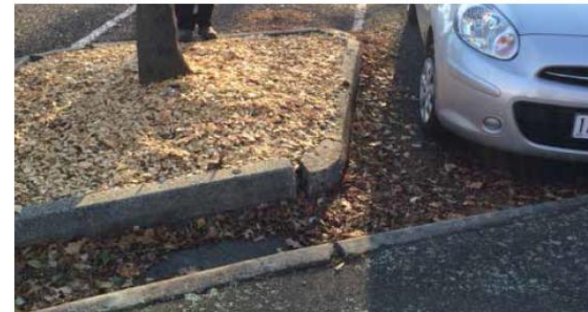
'Island' around tree prevents entry of water from the adjoining road, restricting passive irrigation and limiting soil moisture
