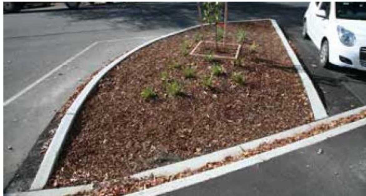
'Island' around tree prevents entry of water from the adjoining road, restricting passive irrigation and limiting soil moisture
