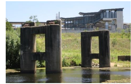
Heritage bridge structure across Georges River
