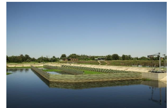
Existing treatment ponds at Liverpool Recycled Water Plant
