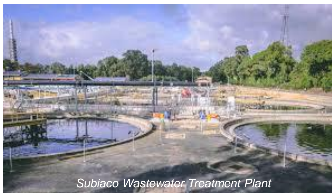
Subiaco Wastewater Treatment Plant
