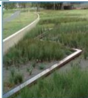
Raingardens in park water and filter pollutants
