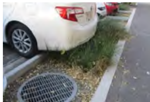
Vehicle and pedestrian damage – impacts vegetation health and causes compaction
