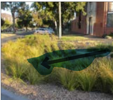
Batter slopes serve a purpose for safety, but need to be factored into design – in this case, the outlet level relative to batter slopes allows only very minimal flow distribution
