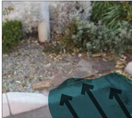
No drop down into biofilter – flow cannot easily enter
