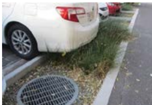
Vehicle and pedestrian damage – impacts vegetation health and causes compaction
