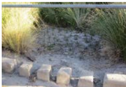
Plant die-back near inlet – may indicate high inflow velocities, sediment accumulation or poor species selection
