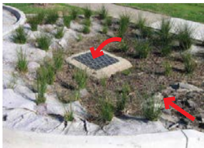
Figure 20. A side entry pit downstream of a biofiltration tree pit accepts high flows that bypass the tree pit (left) while a grated inlet pit close to the inlet of a biofiltration basin conveys above-design flows to the conventional drainage network (right).
