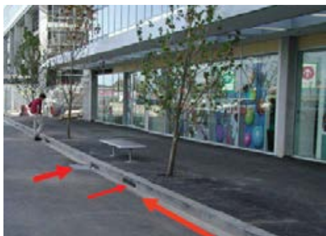
Figure 20. A side entry pit downstream of a biofiltration tree pit accepts high flows that bypass the tree pit (left) while a grated inlet pit close to the inlet of a biofiltration basin conveys above-design flows to the conventional drainage network (right).
