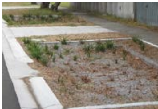
Plant die-back – severely reduces treatment efficiency and leaves media vulnerable to erosion
