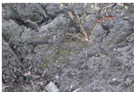
Clogging – build up of fine sediments, moss or plant litter on the surface reduces infiltration and treatment
