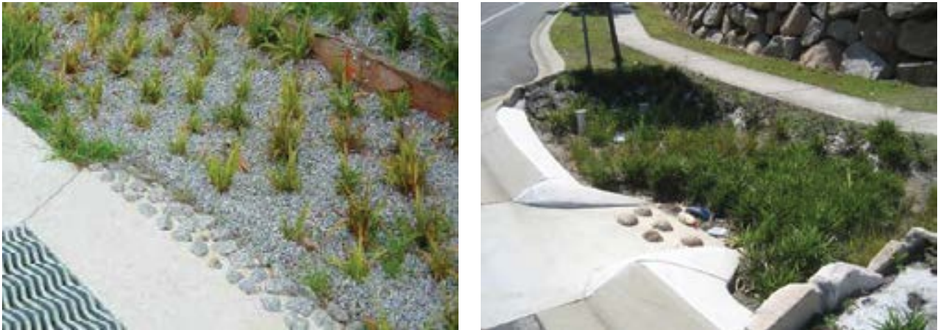
Figure 18. A rock apron (left) and dense vegetation (right) at the inlet to a biofilter can be used reduce flow velocities and prevent scour and erosion damage.
