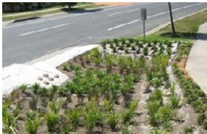
Figure 1. Biofiltration basin at Saturn Crescent, October 2006.
