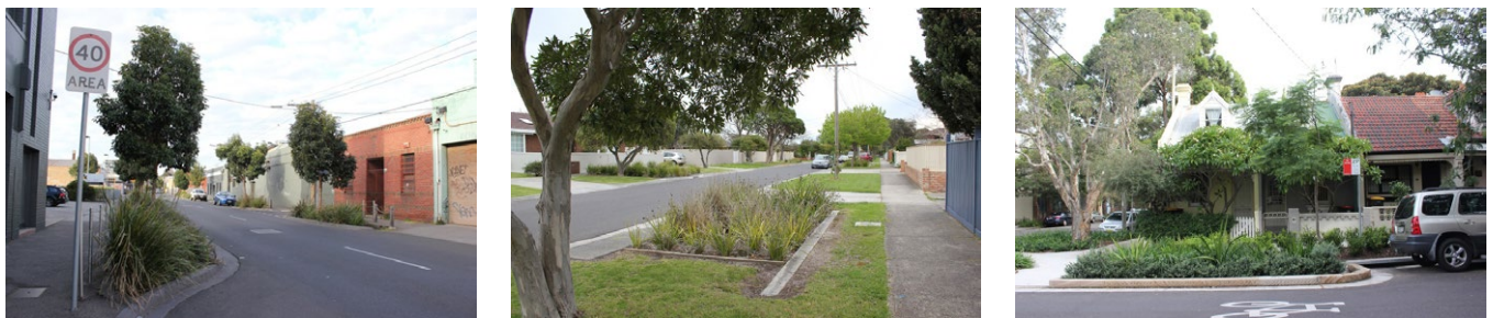
Figure 33. Design of a raingarden should reflect its context, including land use, predominant architectural style and plant selection in the surrounding gardens and streetscape. Photos supplied by M. Dobbie, Monash University
