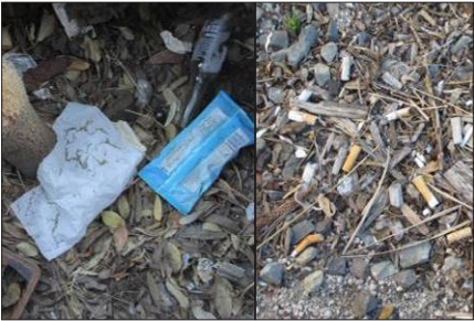
Litter accumulation (anthropogenic and organic) – unsightly and can hinder flow paths and infiltration
