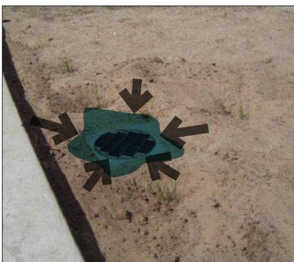
Overfilling with media – reduces or prevents ponding in the ponding zone and reduces treatment capacity
