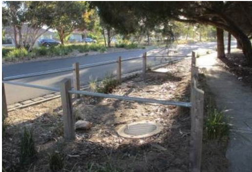
Widespread plant loss or die-back – can indicate too much or too little water, or poor filter function
