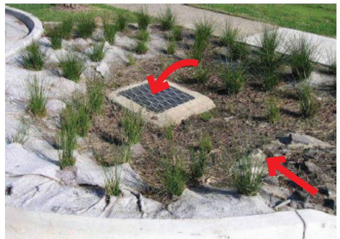
Figure 20. A side entry pit downstream of a biofiltration tree pit accepts high flows that bypass the tree pit (left) while a grated inlet pit close to the inlet of a biofiltration basin conveys above-design flows to the conventional drainage network (right).
