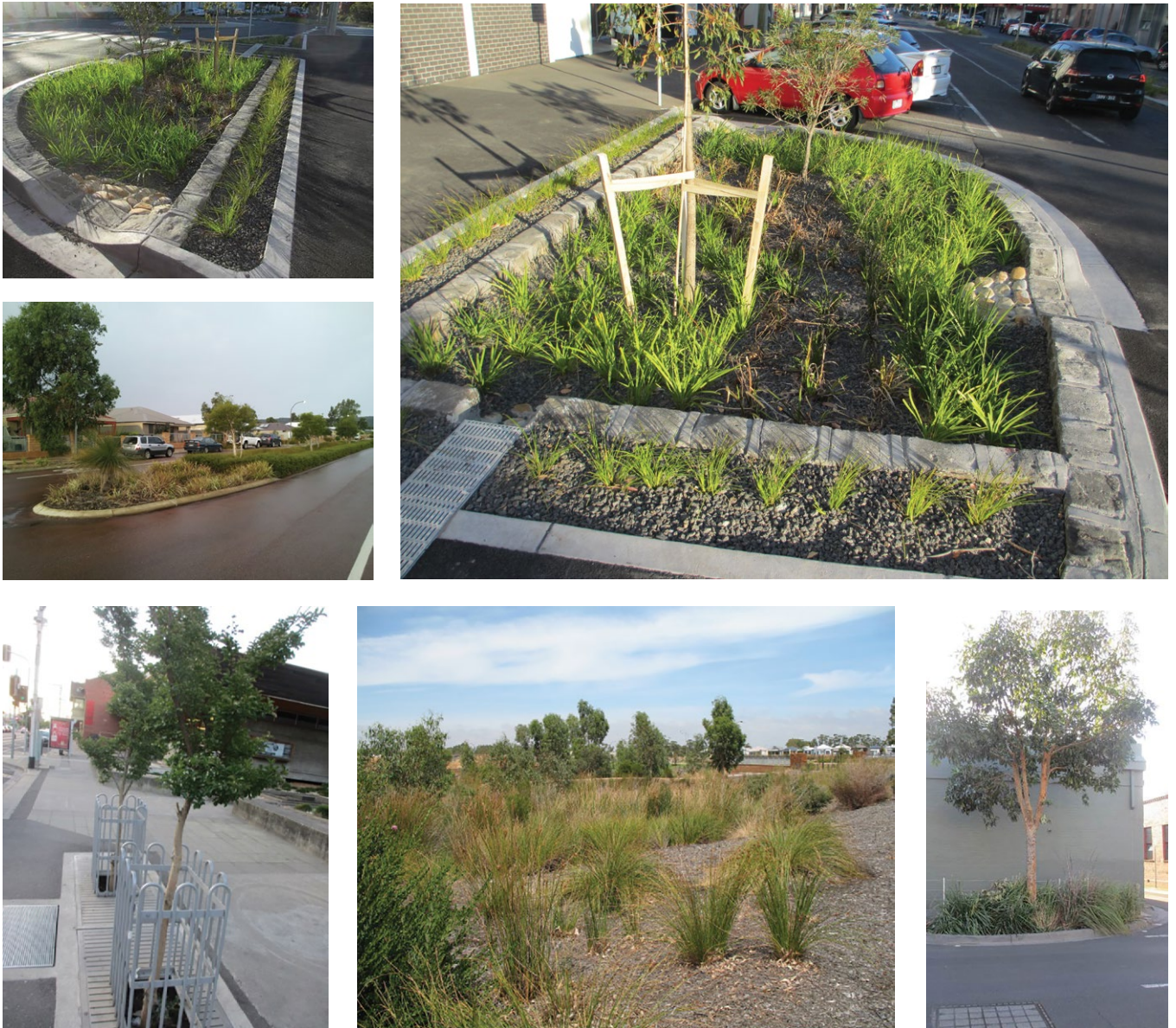
Figure 2. Examples of stormwater biofilters, which can vary widely in their scale, appearance and design to suit treatment objectives and local site conditions. Photos supplied by Krish Seewraj and Antonietta Torre, Department of Water and Emily Payne, Monash University
