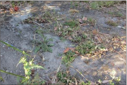
Weeds – unsightly and can reduce treatment capacity
