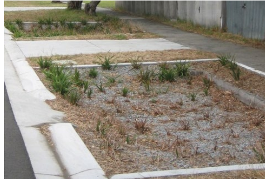
Plant die-back – severely reduces treatment efficiency and leaves media vulnerable to erosion
