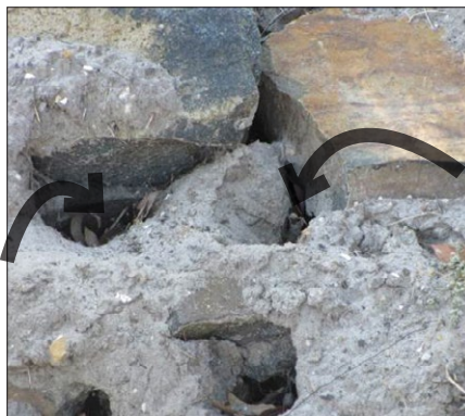
Good hydraulic design, flow management during construction and establishment, and effective sealing is important to prevent erosion and short-circuiting
