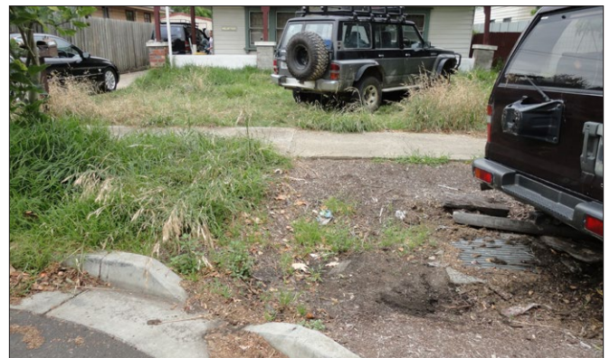
Figure 39. Vehicle damage to a biofilter – frequent parking on top of the system has compacted the media and left it devoid of vegetation. Photo courtesy of Mohammed Al-Ameri, Monash University.
