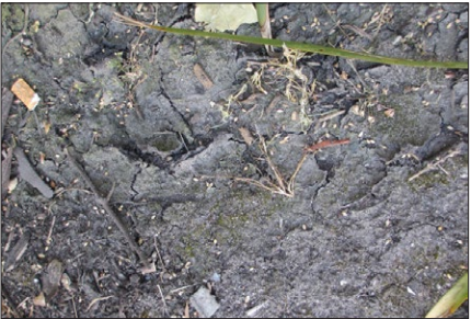
Clogging – build up of fine sediments, moss or plant litter on the surface reduces infiltration and treatment capacity
