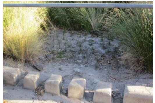
Plant die-back near inlet – may indicate high inflow velocities, sediment accumulation or poor species selection
