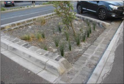
Poor vegetation spread – may be due to use of rock mulch
