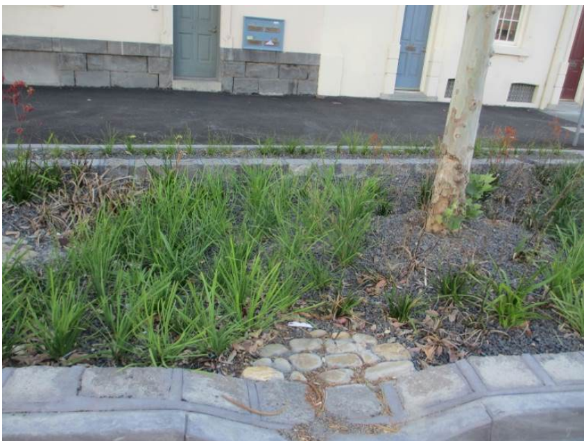
Figure 31. Trees planted on elevated mounds within biofilters (City of Port Phillip)
