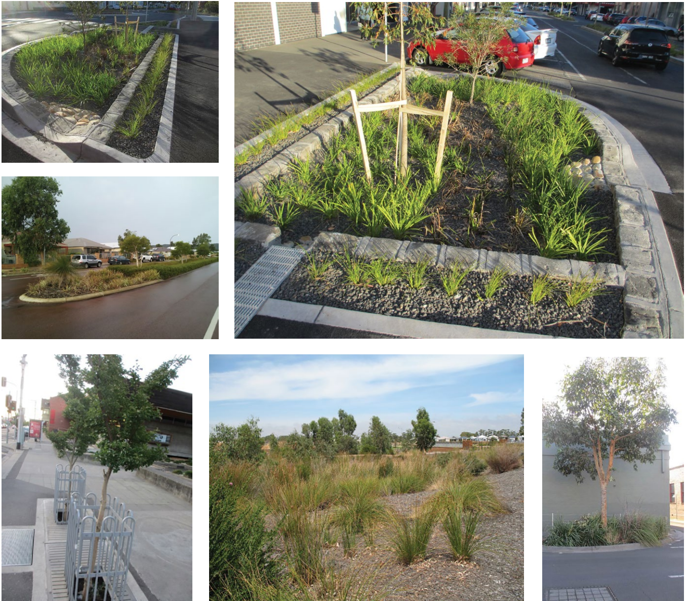
Figure 2. Examples of stormwater biofilters, which can vary widely in their scale, appearance and design to suit treatment objectives and local site conditions. Photos supplied by Krish Seewraj and Antonietta Torre, Department of Water and Emily Payne, Monash University
