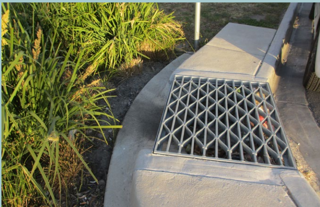
A wide bench area at kerb height provides a safe zone for vehicle drivers and passengers to access kerbside parking
