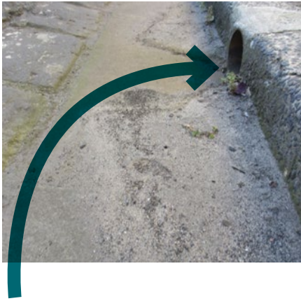
Sediment management: high risk of sediment washing into biofilter during construction in catchment
