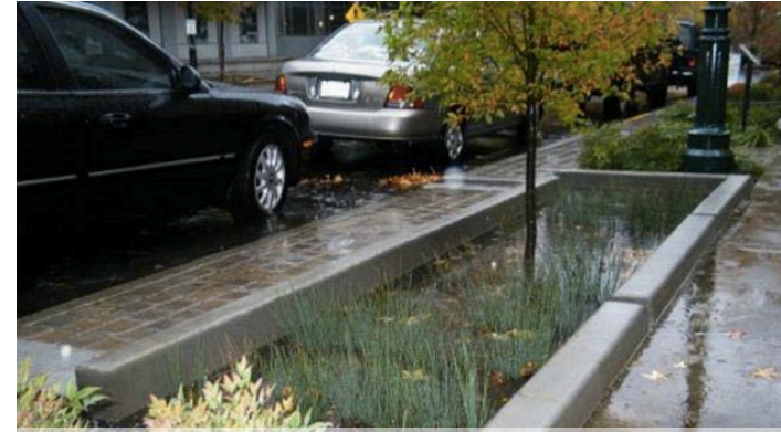
Stormwater planter boxes, SW 12th Avenue, Portland Oregon (UWA and City of Canning, 2016)
