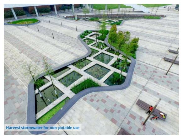
Biofilters are incorporated into the road verge to treat stormwater and detain peak flow.
