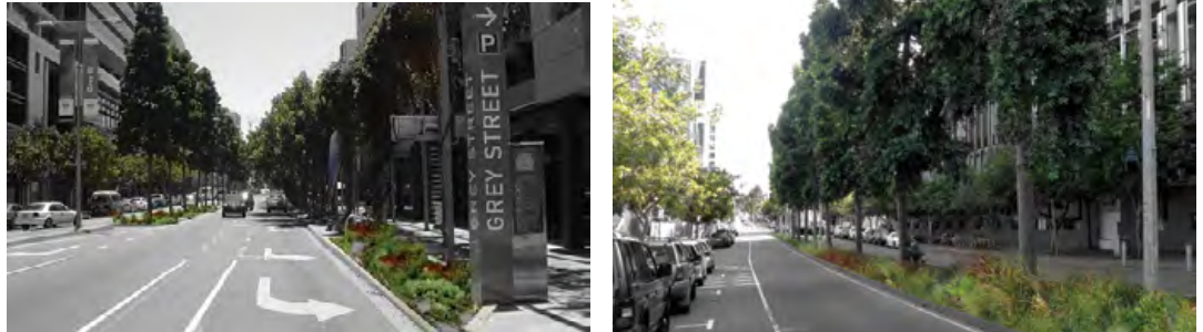
Figure 16 Median strip raingardens are one tool to create a self-irrigating, green street network that extends the benefits of the Parklands deeper into South Bank.
