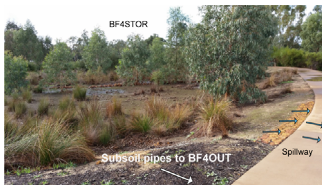
Figure 6: The dry bioretention basin, BF4.
