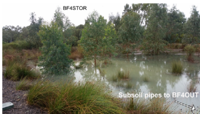
Figure 5: The bioretention basin with standing water.
