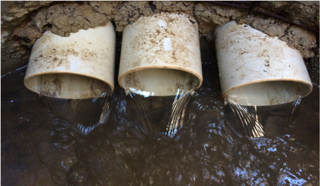
Figure 53: Event on 22 July at bioretention basin outflow (BF4OUT). Discharge from subsurface pipes at a flow rate of 12 L/s. Source D. Sidoti (2015).
