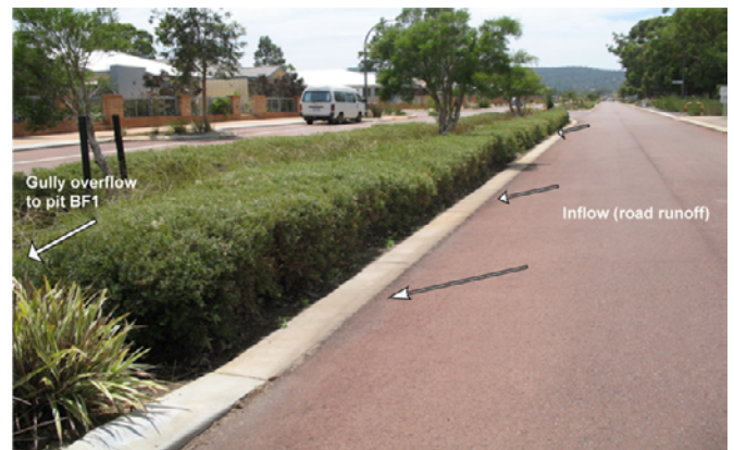
Figure 2: Raingarden comprising vegetated swale and flush kerb for sheet inflow. Arrows indicate flow direction.
