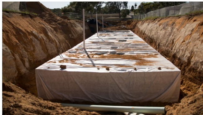
Construction of the storage cells under the sump landscape (Credit: Josh Byrne & Associates)
