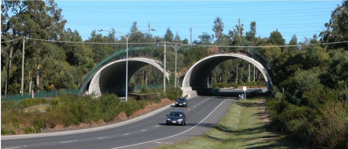
A vegetated overpass providing safe passage for wildlife over Compton Rd, Brisbane. A rope ladder providing passage for possums is shown in the foreground. Photo: Darryl Jones
