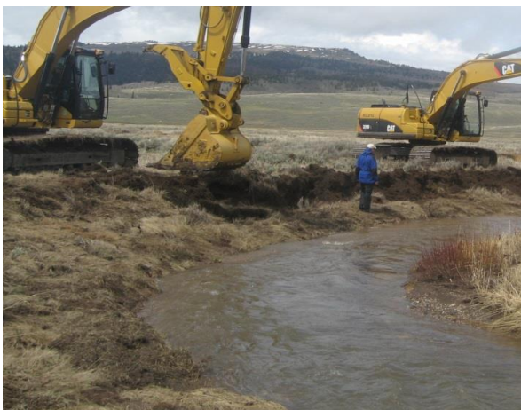
Excavation of a floodplain terrace. Taken from Boyd (2015)
