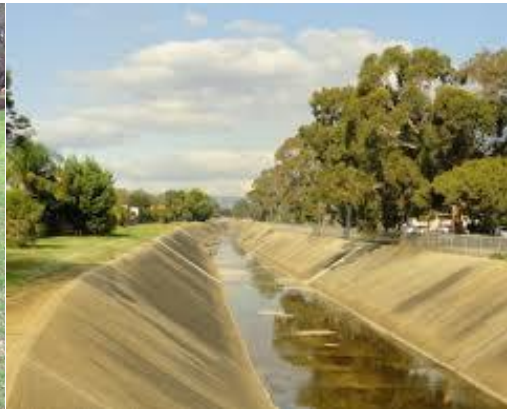
Concrete-lined trapezoidal drain Adelaide. Photo: unknown source
