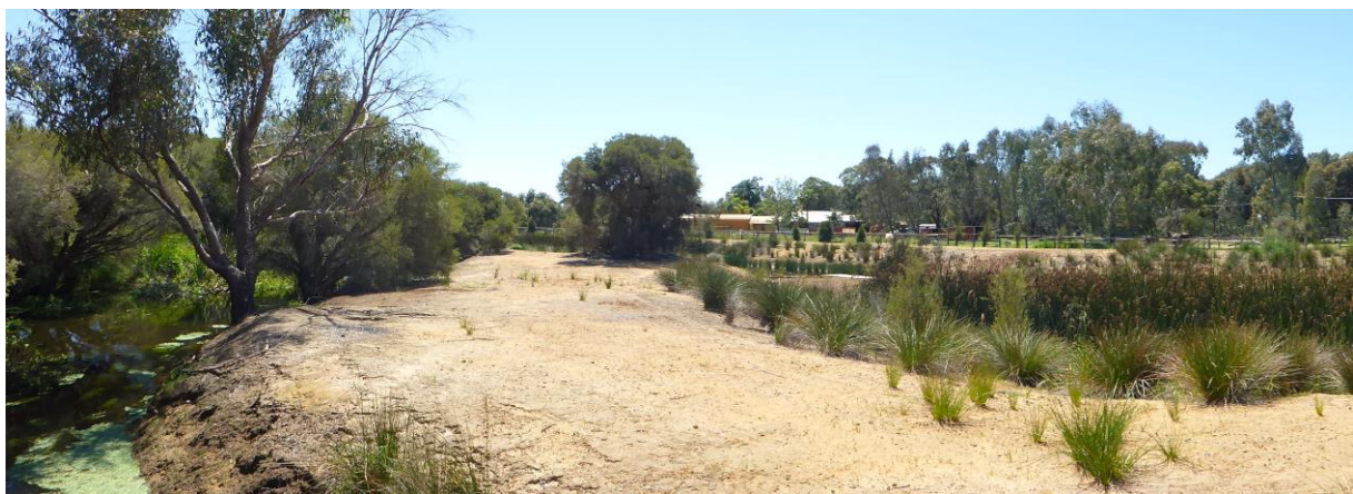
A wetland biofiltration basin adjacent to a natural creek line in Perth that treats stormwater before it enters the river and also receives high flows, moderate downstream flows during floods. Photo: Belinda Quinton
