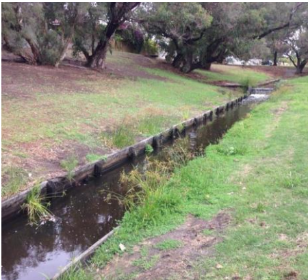
Wood revetment and channelisation of Bennet Brook drain, Perth. Photo: Leah Beesley
