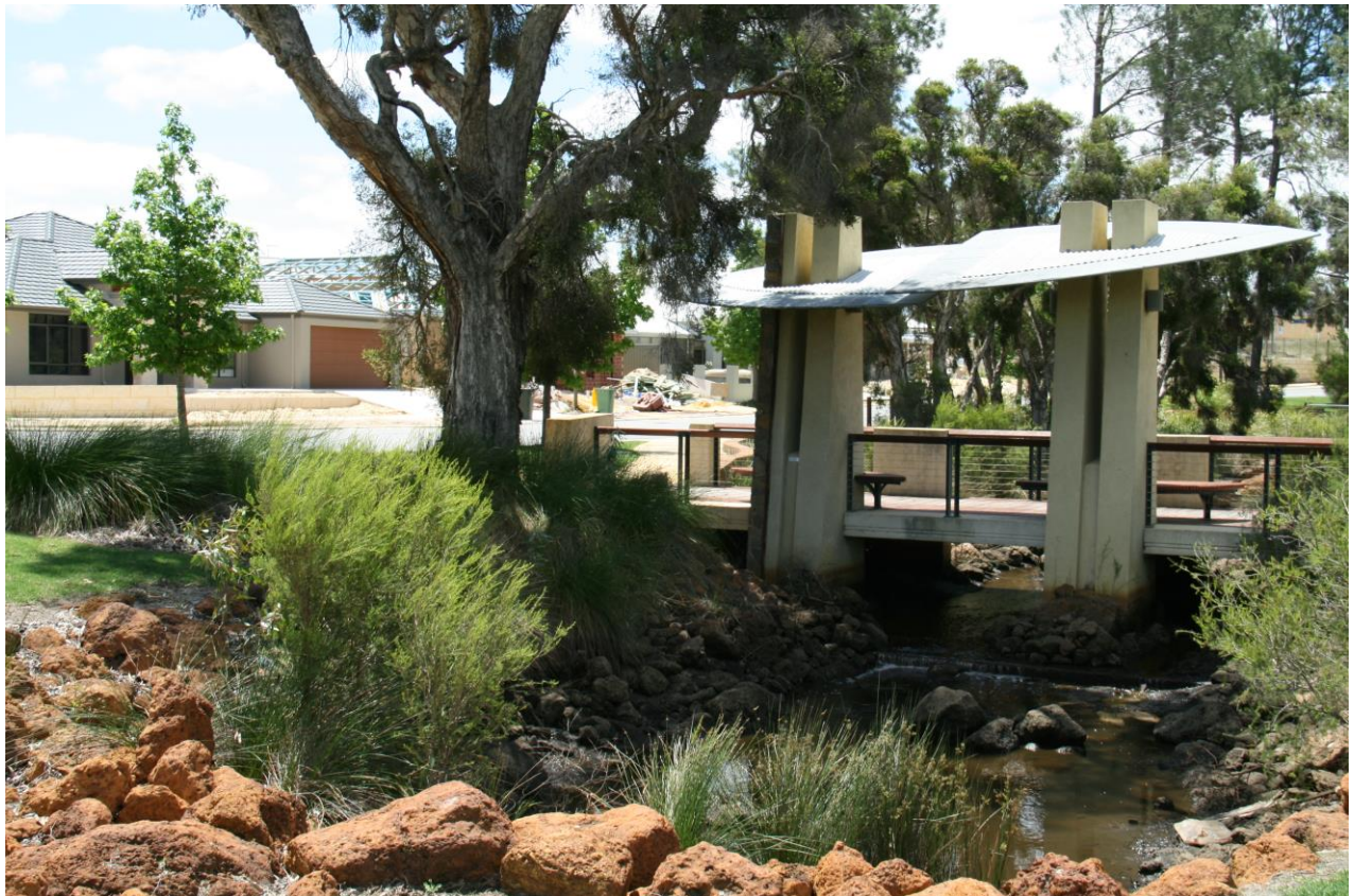
Artificial structures, such as viewing platforms, can create some stream shading, albeit very limited. Photo: Belinda Quinton
