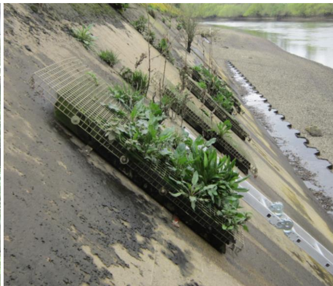
Wall box attached to concrete lined channel, Thames River, London. Photo: Robert Francis
