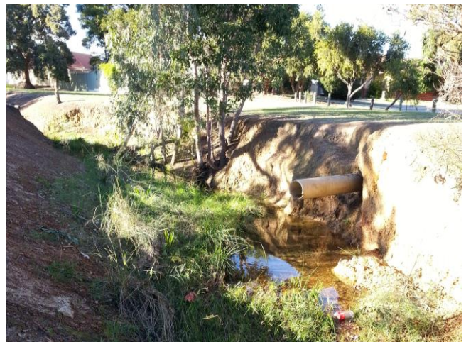
The direct piping of stormwater to a stream channel, Armadale, Perth. Photo: Leah Beesley
