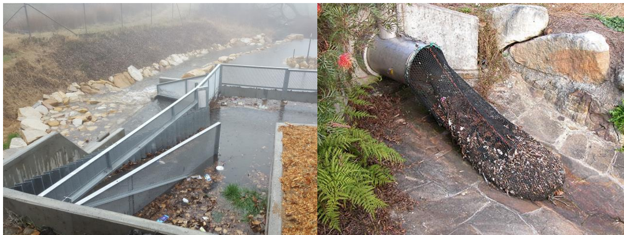
Leaves trapped in a GPT Blue Mountains. Photo: Geoffrey Smith Leaves trapped in a GPT Hornsby Shire, NSW. Photo: unknown
