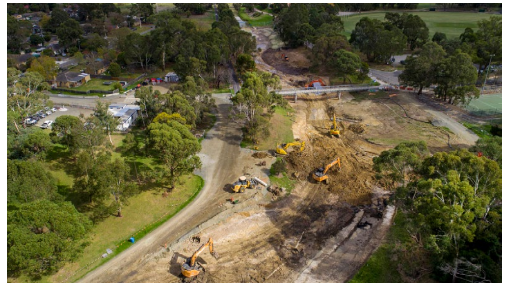
Drone footage during construction, daylighting 830m of Dandenong Creek (image courtesy of Melbourne Water)
