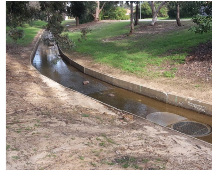
Existing urban drain from which flows are harvested and injected into the underground aquifer
