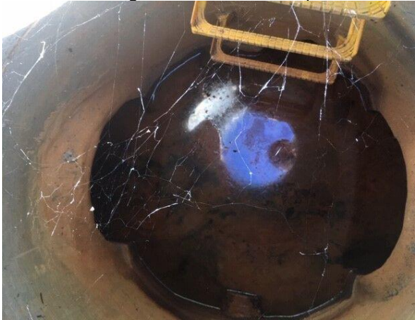
Coralvine Grange and Roselea Blvd pit
