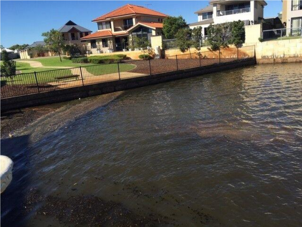
Sediment accumulation at the Inflow northern end: lake level at 10.25 m (March 28 2019)
