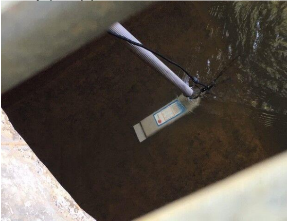
Karrinyup Rd pipe: flow measurement
