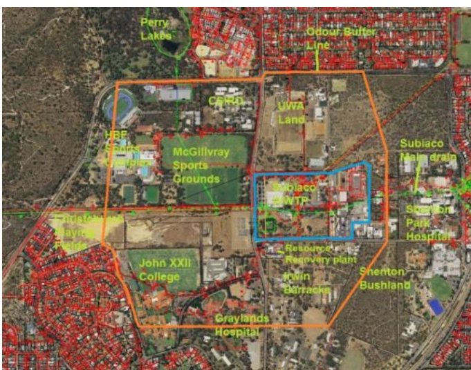
Figure 1: Subiaco Wastewater Treatment Plant (blue) and odour buffer zone (orange). Source: Water Corporation
