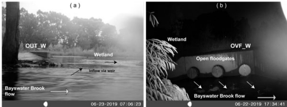
Figure 8 Camera stills used in flow monitoring at ESBS Outlet and Overflow: a) water exchange between Bayswater Brook and the wetland via weir structure, and b) discharge from wetland to Bayswater Brook at OVF_W under high water levels (note floodgates upward allowing discharge).
