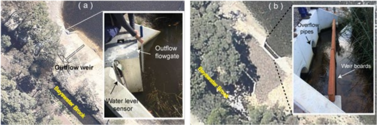
Figure 4 Outflow structures controlling discharge from ESBS; a) main Outflow point and associated surface overflow weir, b) Overflow structure and wooden boards weir used in management actions to control water levels in the wetland.
