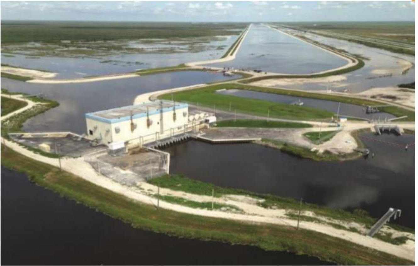
Figure E-1: Flow Equalization Basin in Palm Beach County, Florida, flowing into a contributed wetland. Source: SFWMD (n.d.-a)
