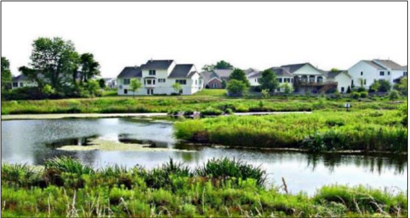
Figure E2 Wet pond in Virginia, within the Chesapeake Bay Watershed Source: Chesapeake Stormwater Network (2018)
