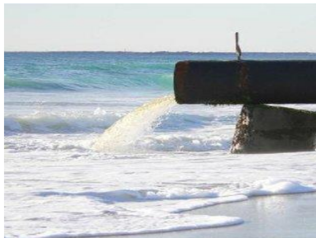
Figure 2: Stormwater entering the ocean (need to replace)
