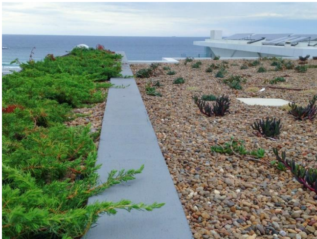
Figure 3: Green roof in Bondi (Atlantis Aurora) – need replacement
