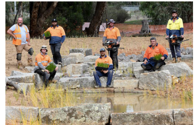
↑ Djandak team members at Koomba Street's new project healing storm water before it flows into the Bendigo Creek. Picture: NONI HYETT
