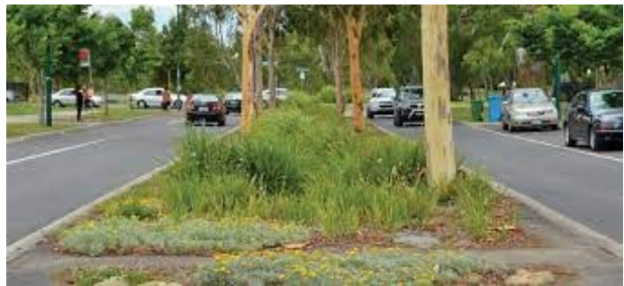
Figure 32: Swale between two roads in Lyndhurst.
