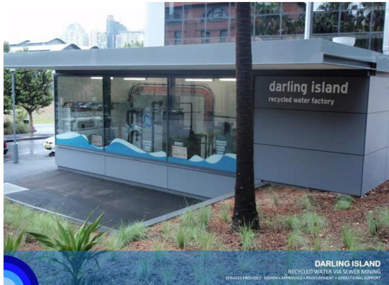
Figure 19: Darling Island Wastewater Treatment and Recycling Facility.
