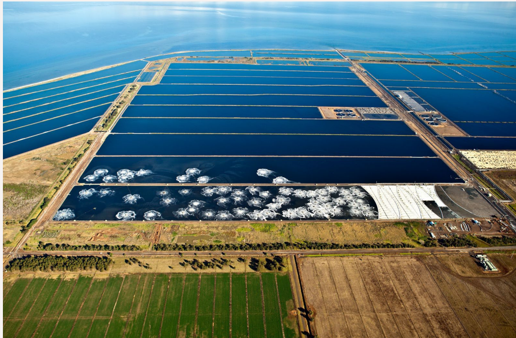
Figure 33: The Western Treatment Plant.
