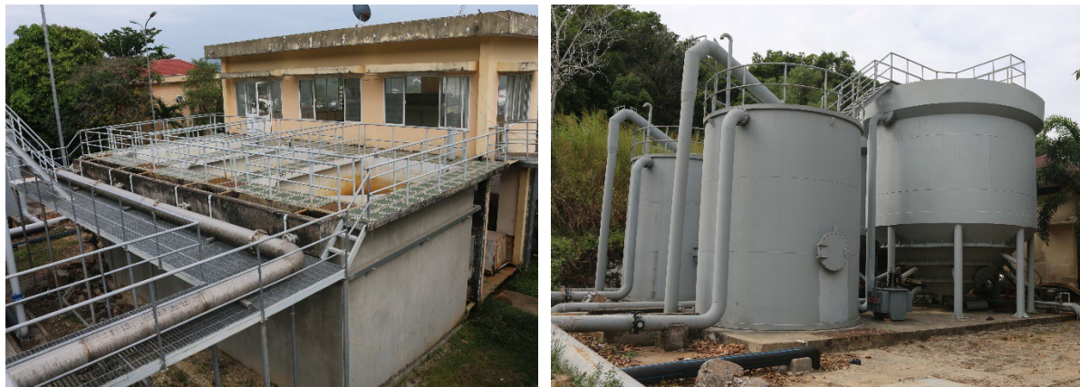
Figure 5: Existing Duong Dong WSS.
