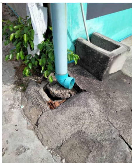
Figure 7: Leaves and trash partially blocking a drain (left) and unconnected downpipe (right). Source: Project team, December 2020.
