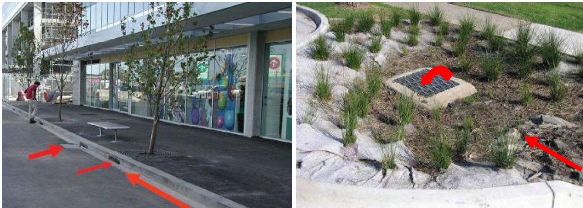
Figure 15. A side entry pit downstream of a biofiltration tree pit accepts high flows that bypass the tree pit (left) while a grated inlet pit close to the inlet of a biofiltration basin conveys above-design flows to the conventional drainage network (right).
