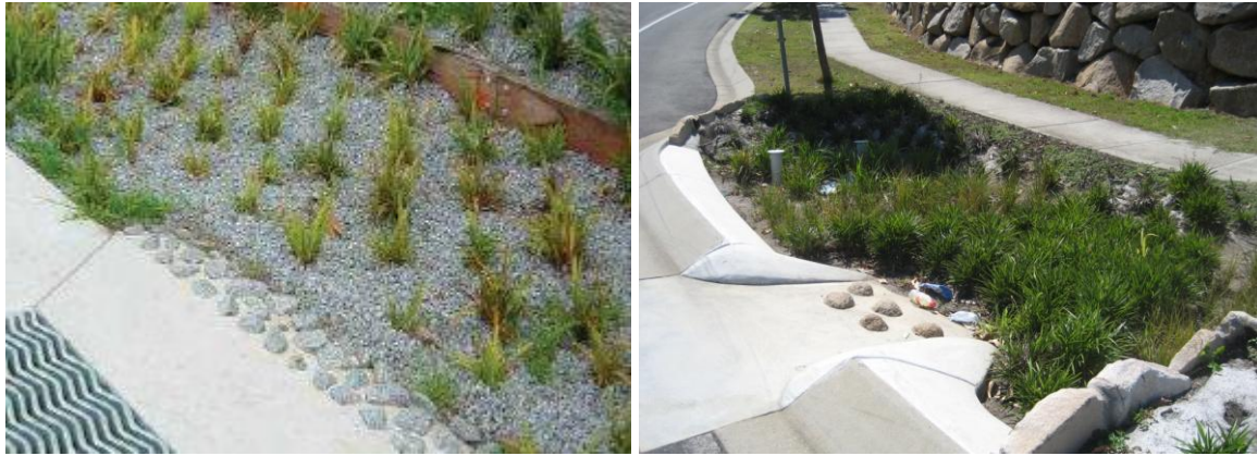
Figure 13. A rock apron (left) and dense vegetation (right) at the inlet to a biofilter can be used reduce flow velocities and prevent scour and erosion damage.
