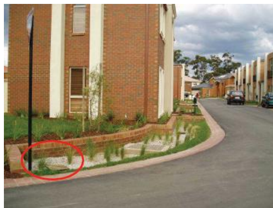
Figure 13. A rock apron (left) and dense vegetation (right) at the inlet to a biofilter can be used reduce flow velocities and prevent scour and erosion damage.
