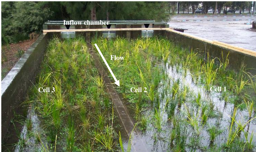
Figure 8. Monash University carpark biofiltration system
