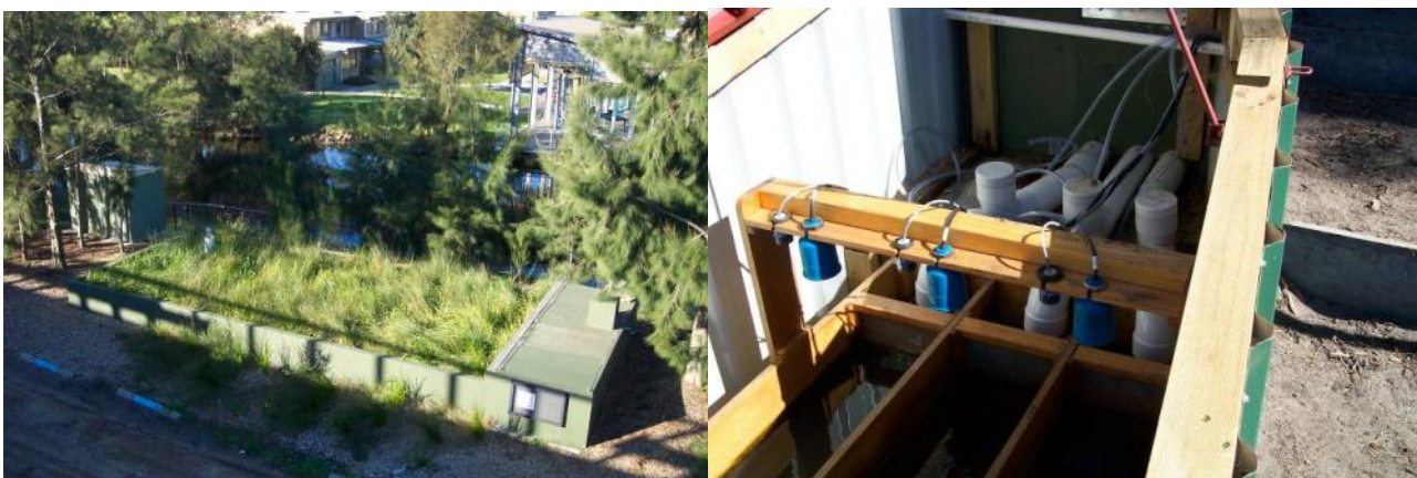
Figure 9. Monash carpark stormwater harvesting system
